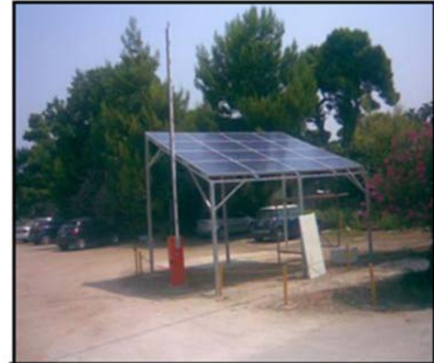
Holiday Camp Meltemi Flexible load: refrigerators of the super market (~15 kW)
