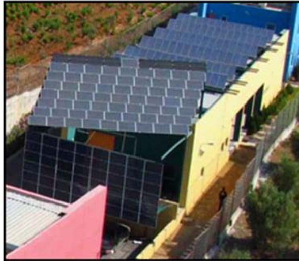
CRES: 22 kW p PV Flexible load: heat pump (61 kW cooling capacity)
