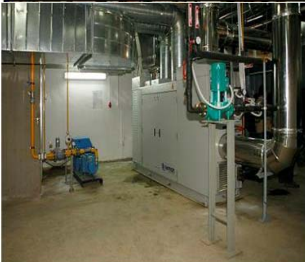
NTUA: CHP 80 kW e Flexible load: cooling system (90 kW electric input)
