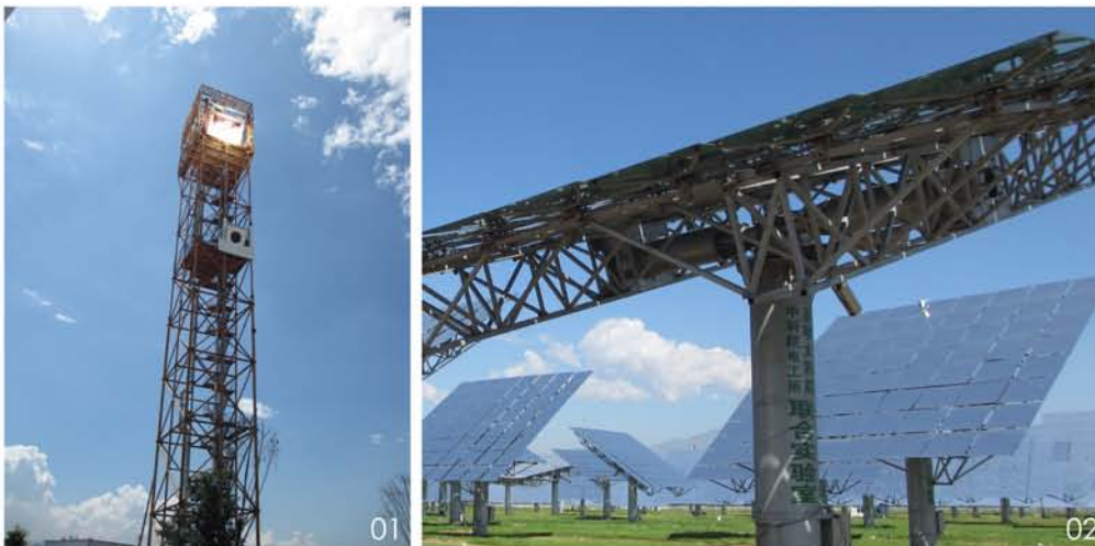
01/02 Beijing Badaling Solar Thermal Power Plant
